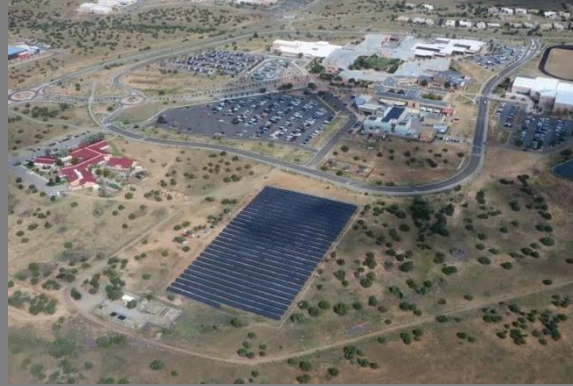
Santa Fe Community College 1.5MW Solar array
